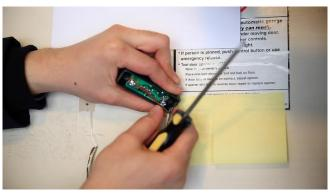
5.1.1.4 The remaining wires will go into the Garage Door Control Button
